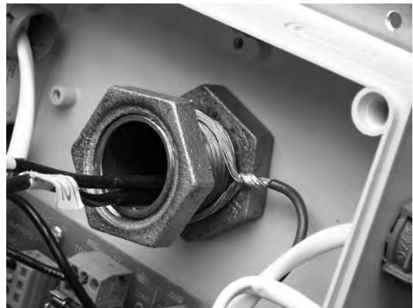
Figure 9: Mounting Sequence, Inside Rear of Fuse Box
