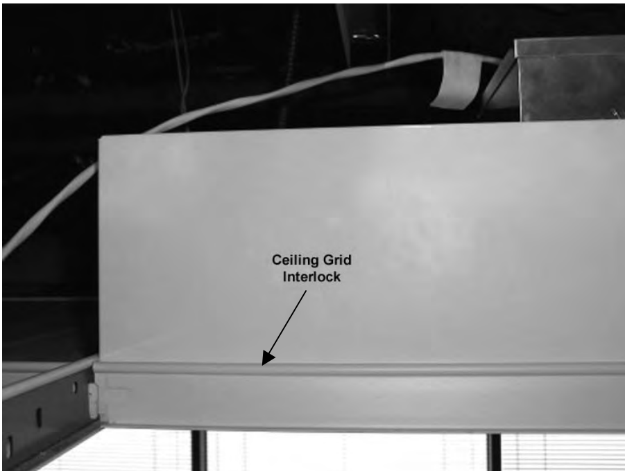
Figure 12: CCT Light box & Grid Supports
