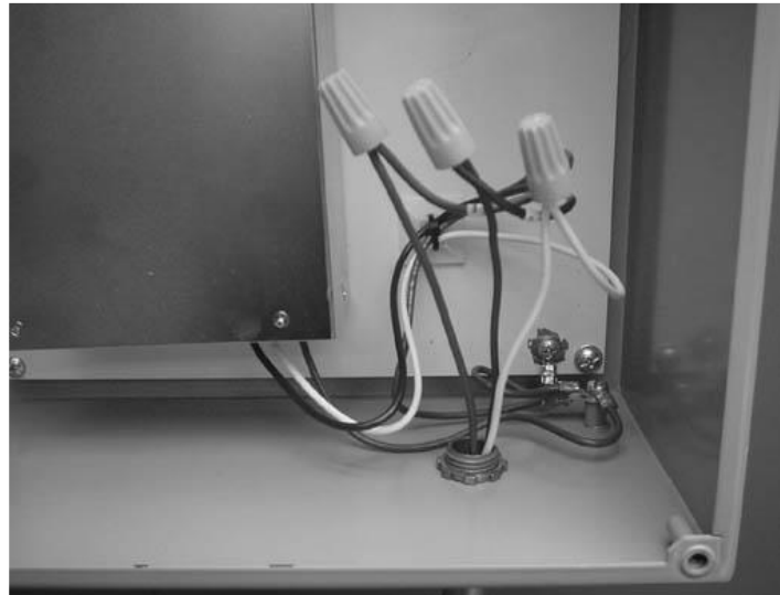
Figure 2: Grounding Post Locations
