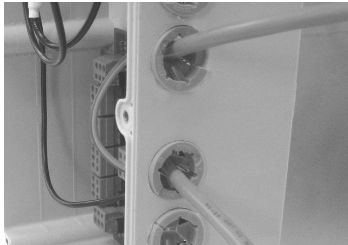
Figure 9: Cable Locking Connector
